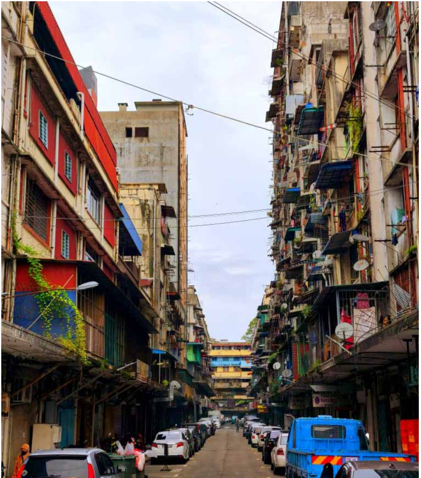
'Little Hong Kong'; combination of residential flats and business on the ground floors (source: author 2025)
