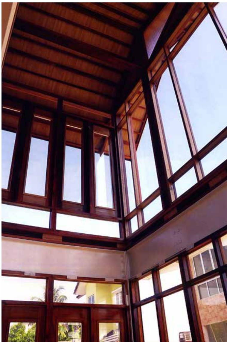
Figure 2: Details of timber framing system on steel beams.
