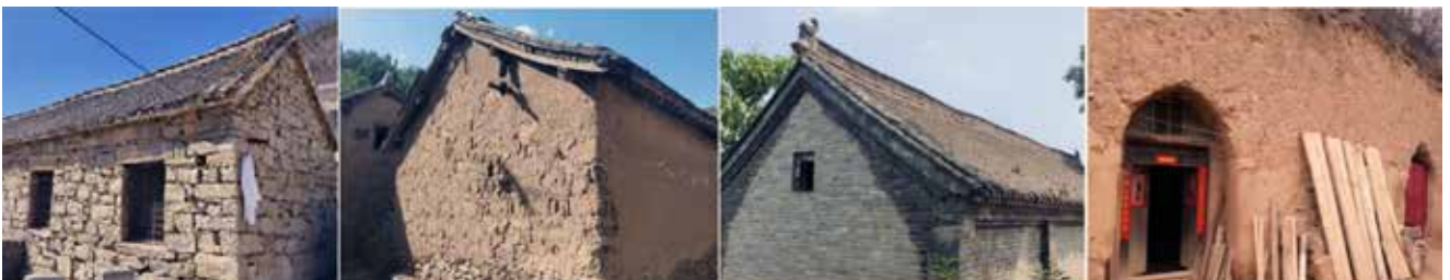
Figure 1: The Main Forms of Vernacular Architecture in Northwest Henan (From Left: Stone Dwellings, Adobe Dwellings, Brick Dwellings and Cave Dwellings)
