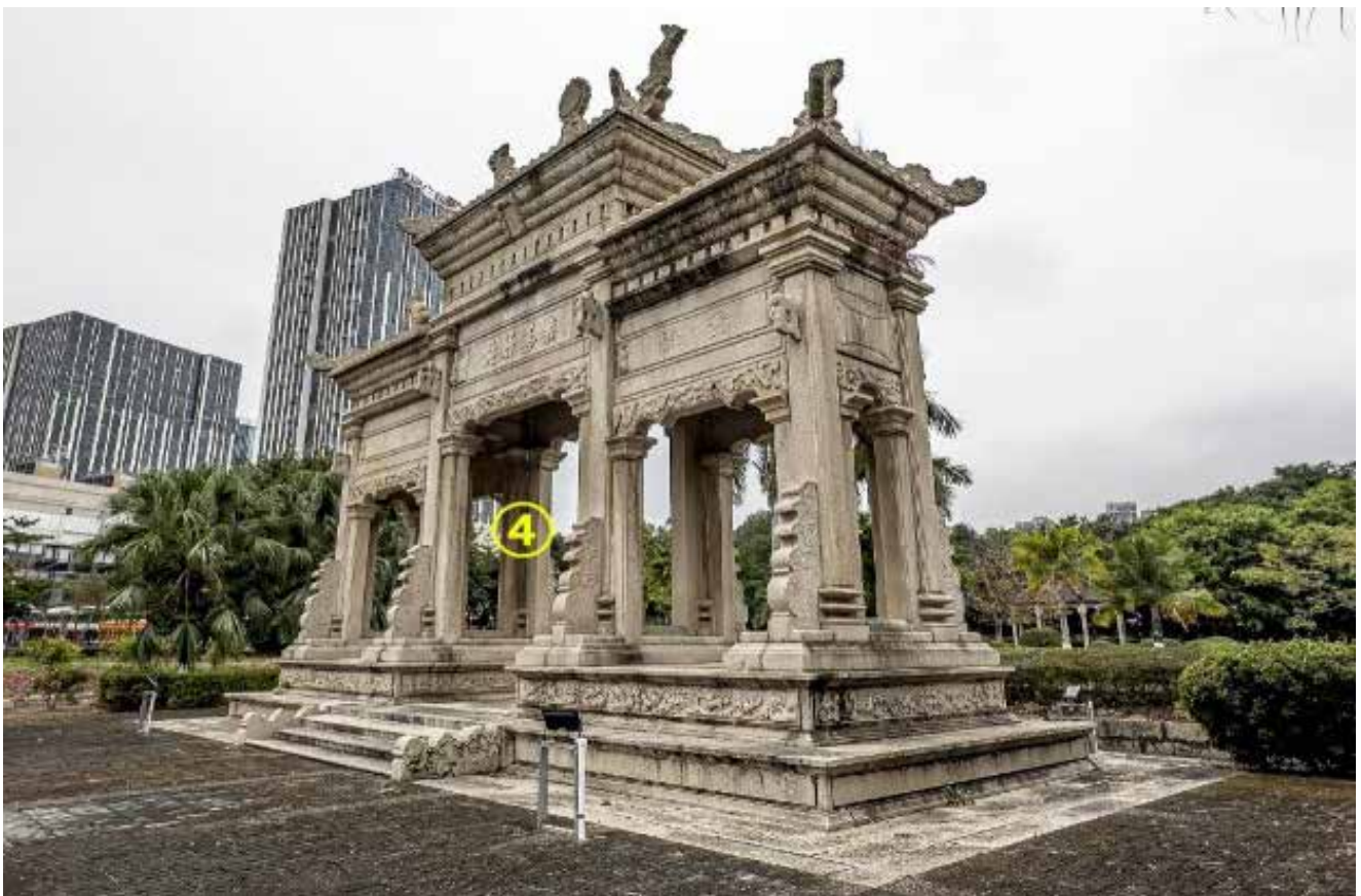
Figure 5: View towards ④.
