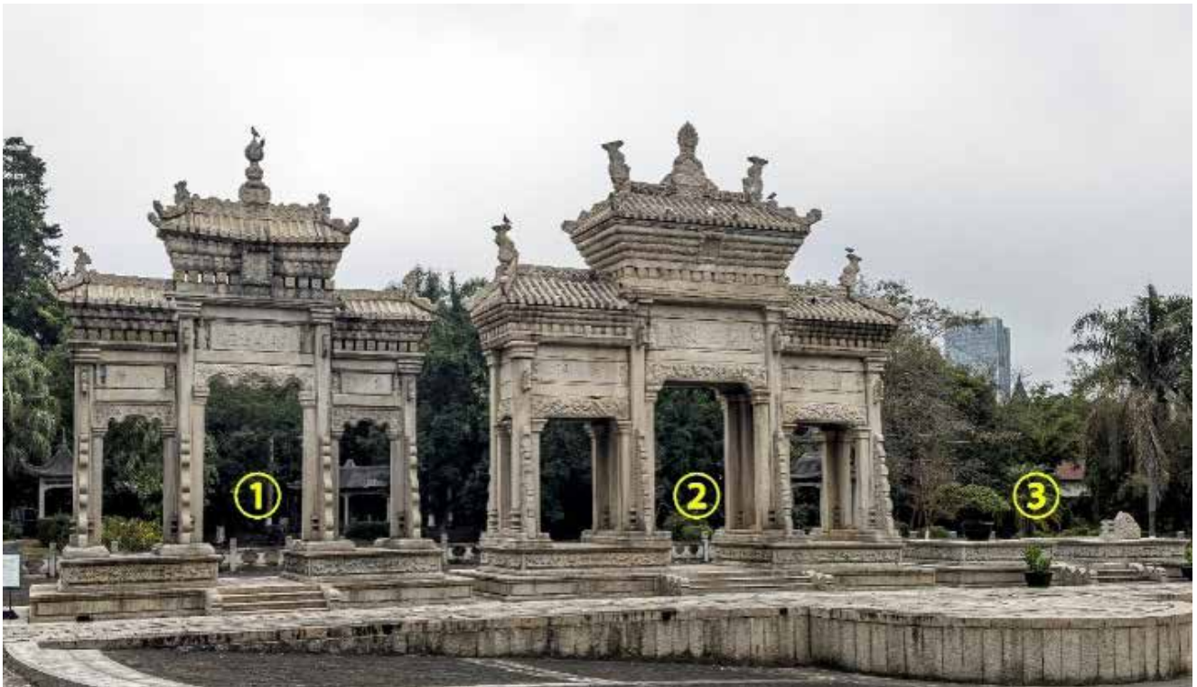
Figure 4: View towards ①-③.
