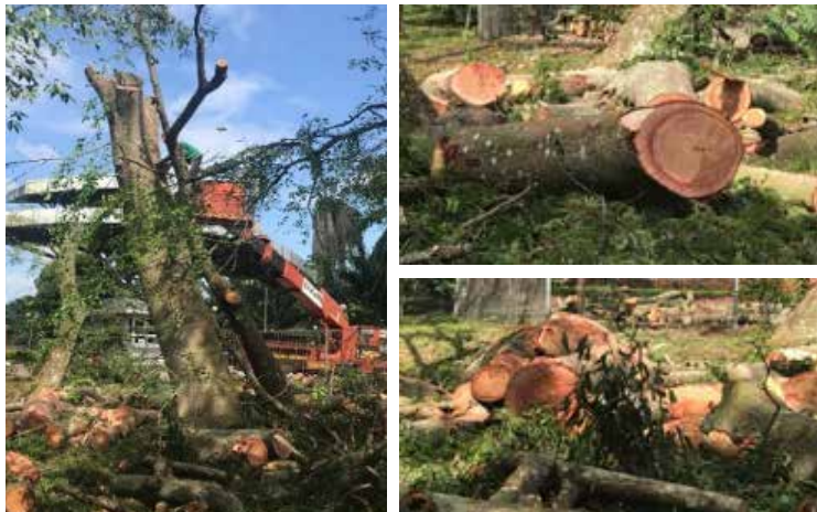
Figure 1: Tree removal for safety reason (Source by authors)
