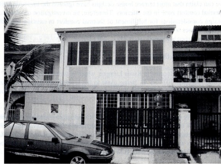
Figure 2: Front facade of the case study building.
